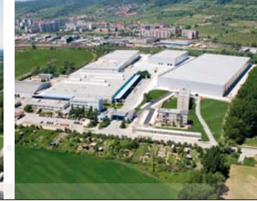
Logistics Center Bratislava – Rača
